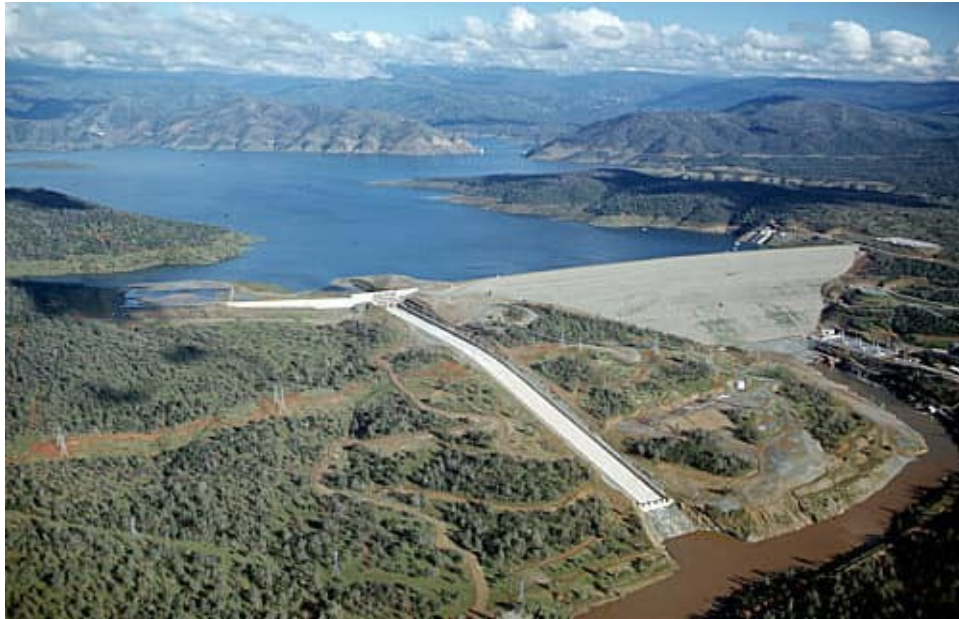
Oroville Dam and Spillway
