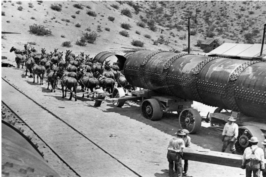
Mule team hauling materials to build the Los Angeles Aqueduct The roadless territory was too tough for the automotive travel of that era
