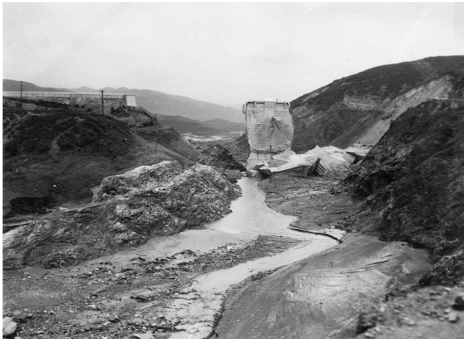
Saint Francis Dam, after its collapse
