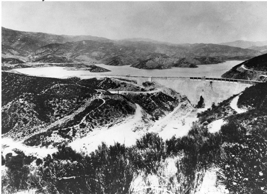
Saint Francis Dam-- shortly before its collapse
