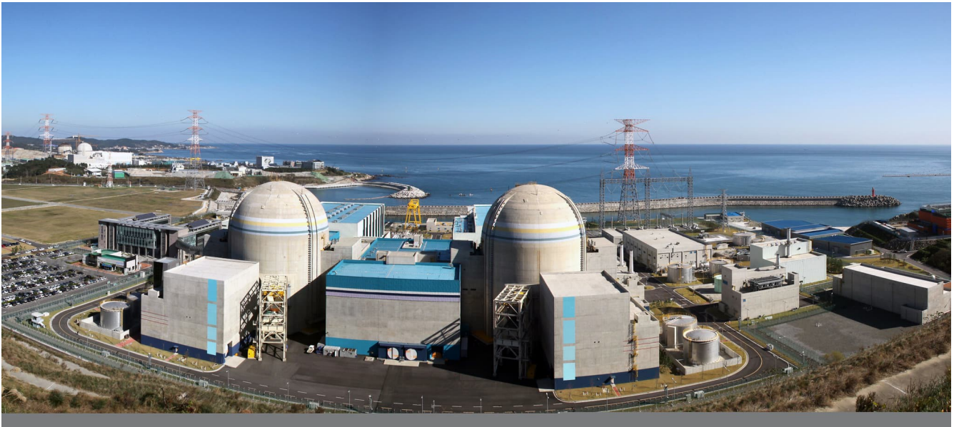
Unit 1-2 of Korea Shin-Kori Nuclear Power Plant. Taken on February 25, 2013. Photo Credit: Korea Shin-Kori NPP / IAEA / Attribution-ShareAlike 2.0 Generic
