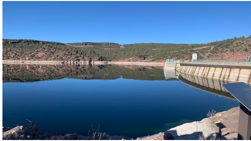
Scenic view of Flaming Gorge Dam in Dutch John, Utah
