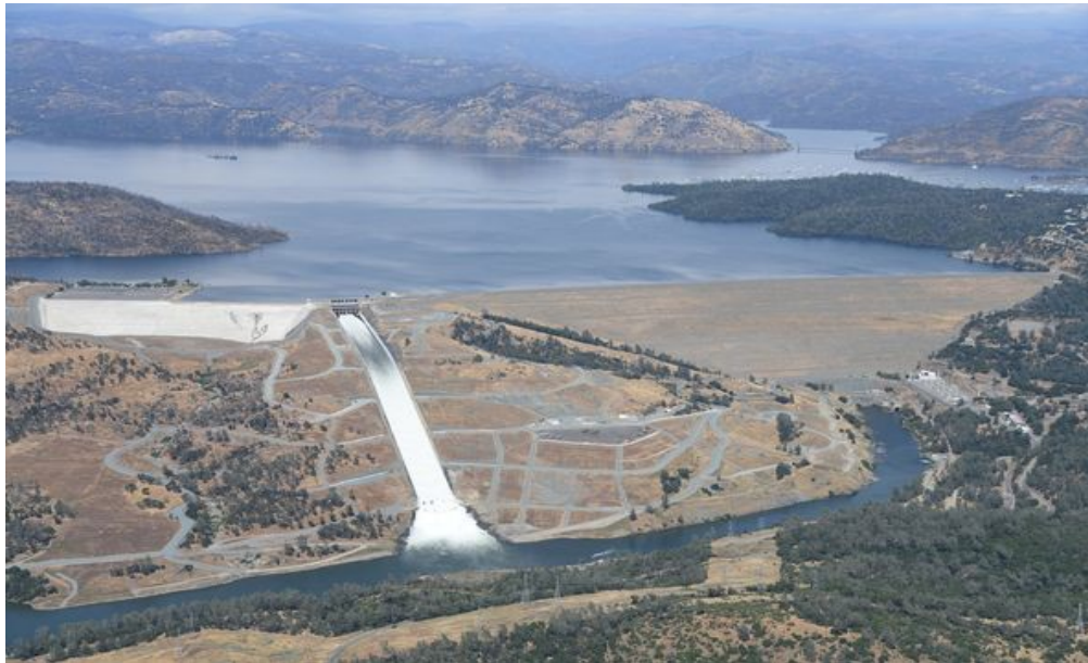
Oroville Dam and Reservoir
