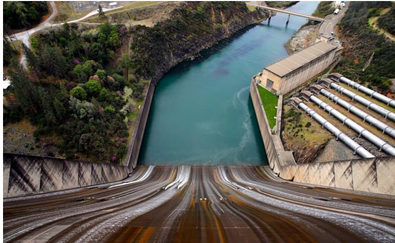
A view down the spillway of the Shasta Dam into the Sacramento River in Shasta Lake, California (Michael Macor/The San Francisco Chronicle via Getty Images)
