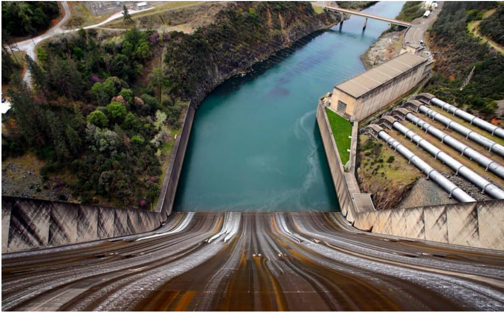
A view down the spillway of the Shasta Dam into the Sacramento River in Shasta Lake, California (Michael Macor/The San Francisco Chronicle via Getty Images)
