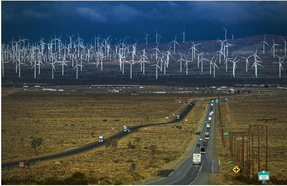
The “scenic beauty” of Biden's Green Energy Policy (See page 8 for article) Wind turbines in the California desert are seen from Highway 58 in 2021. (Irfan Khan / Los Angeles Times)
