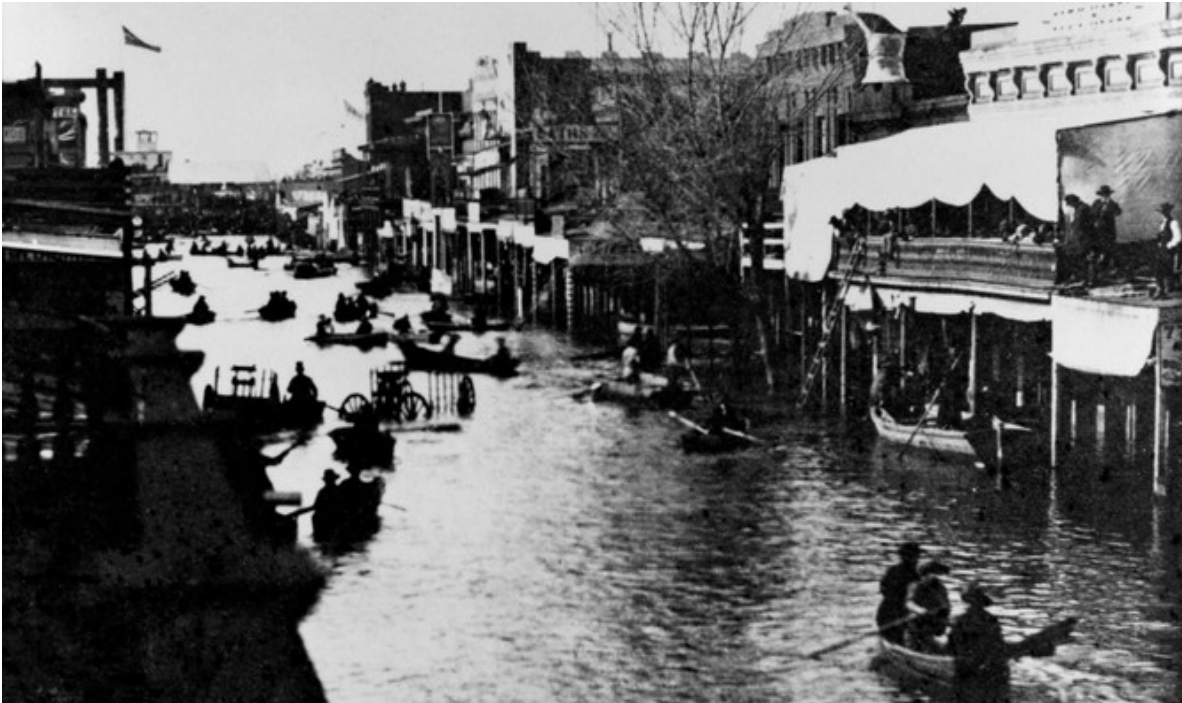
Floodwaters in Sacramento, California in January 1862. (California State Library / FOX Weather)
