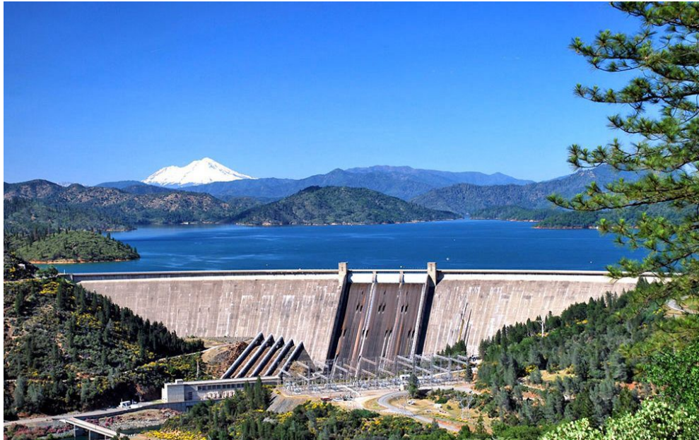
Shasta Dam Raising Project would heighten dam 18.5-feet. (Photo: U.S. Bureau of Reclamation)
