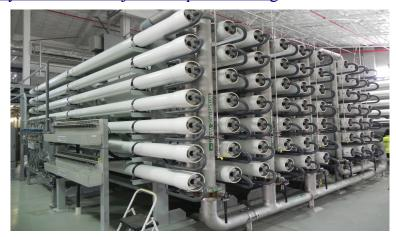
Photograph of a skid of reverse osmosis membranes installed at the Alameda County Water District Newark Desalination Facility. These membranes, installed in 2010, remove salts from brackish groundwater to provide high quality water to local customers.
