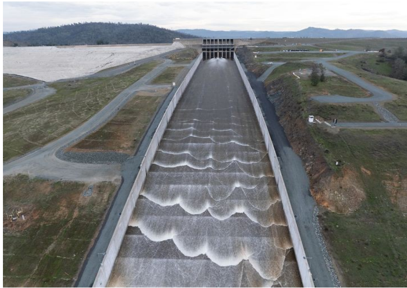
The Oroville Dam's main spillway releasing water from Lake Oroville. The spillway was rebuilt after the devastating collapse in 2017. (Photo credit: California Department of Water Resources)
