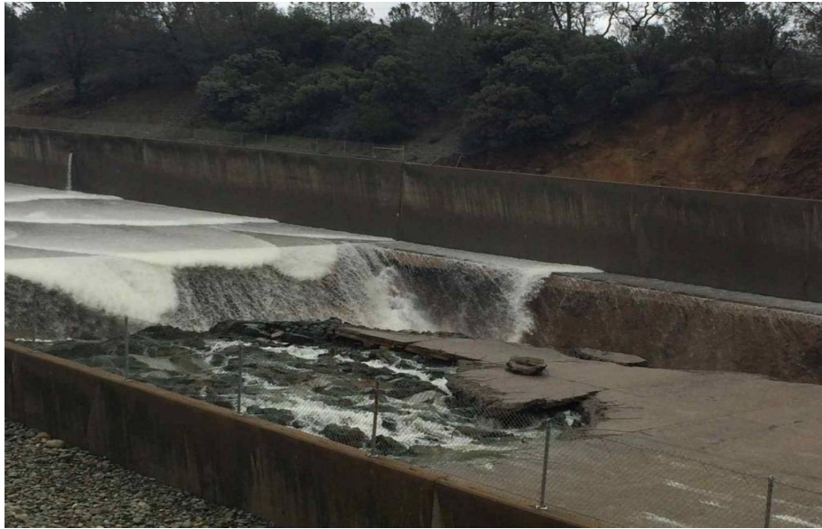
Damage to Oroville Dam's spillway is visible in photo taken after releases were halted Tuesday afternoon. ( Paradise Post via Twitter )
