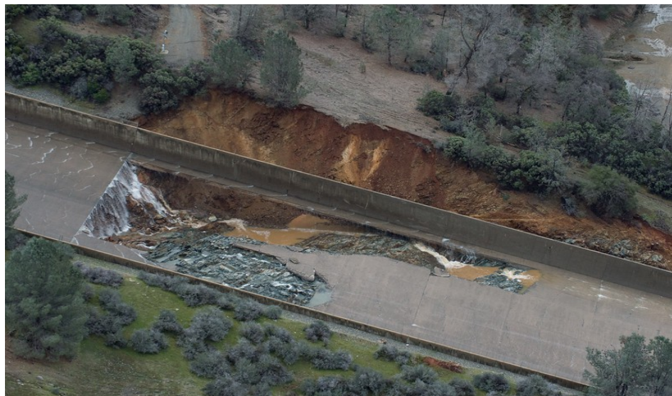
The California Department of Water Resources has suspended flows from the Oroville Dam spillway after a concrete section eroded on the middle section of the spillway. There is no anticipated threat to the dam or the public. DWR engineers are assessing the options to repair the spillway and control the reservoir water level. The Butte County facility is the tallest dam in the United States at 770 feet and is a key part of the State Water Project. Photo taken February 7, 2017.
