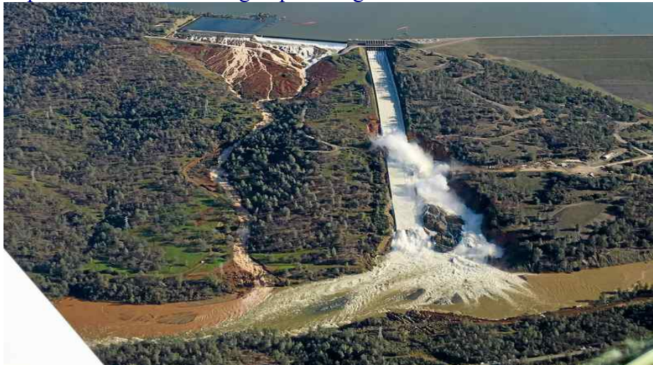
Oroville Dam and spillways
