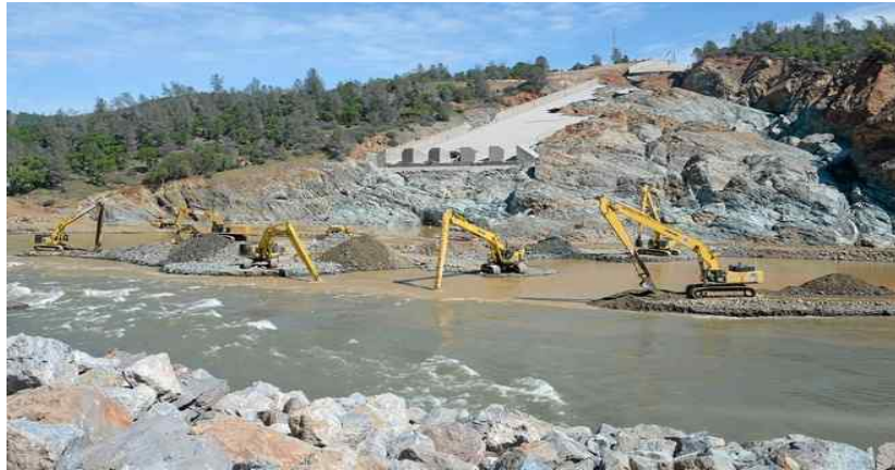
Excavators remove debris from the Diversion Pool below the main Oroville Dam spillway in this photo from March 29. Bill Husa — Mercury-Register
