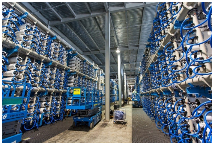
The Carlsbad CA desalination plant
