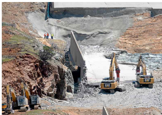
Heavy equipment works Wednesday to break up remaining concrete on the lower part of the damaged main Oroville Dam spillway so a replacement can be constructed. (Bill Husa — Mercury-Register)
