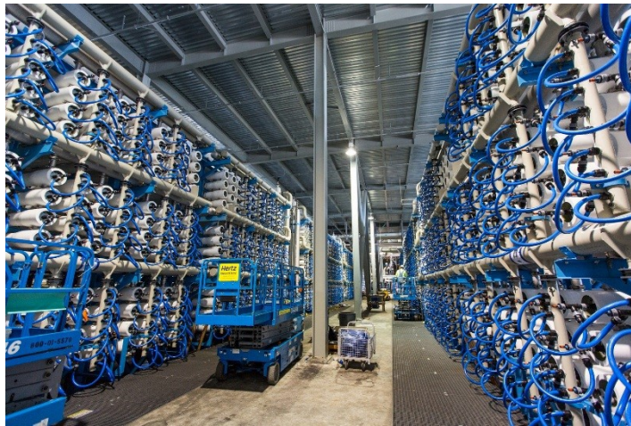
The Carlsbad CA desalination plant
