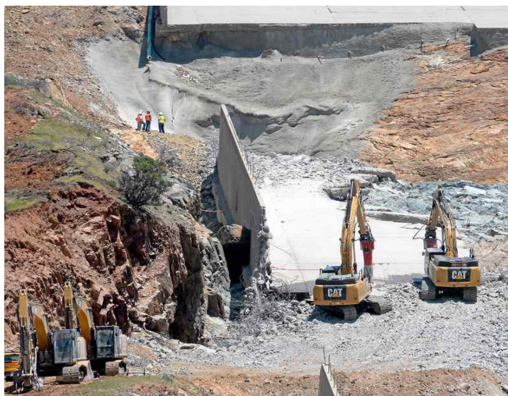
Heavy equipment works Wednesday to break up remaining concrete on the lower part of the damaged main Oroville Dam spillway so a replacement can be constructed. (Bill Husa — Mercury-Register)
