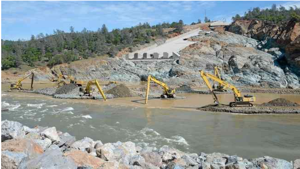
Excavators remove debris from the Diversion Pool below the main Oroville Dam spillway in this photo from March 29. Bill Husa — Mercury-Register
