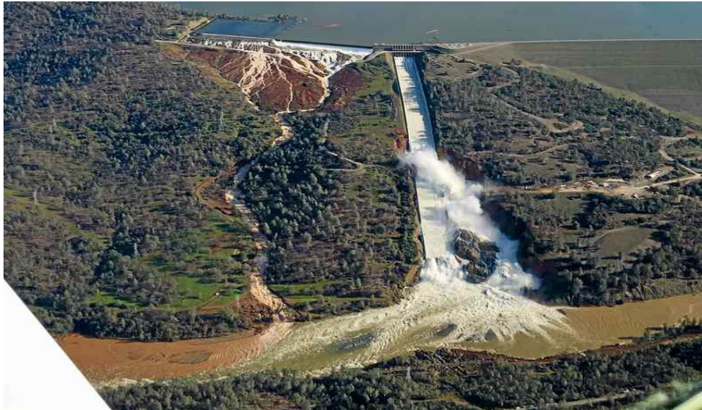
Oroville Dam and spillways
