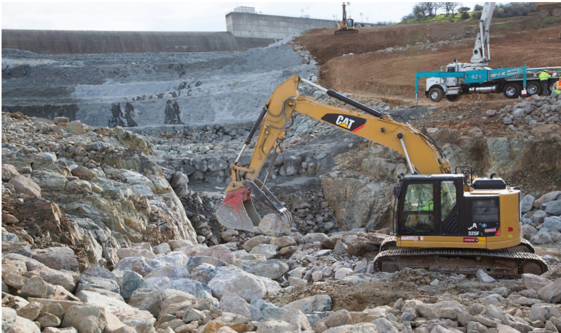
Removing the remains of the damaged spillway
