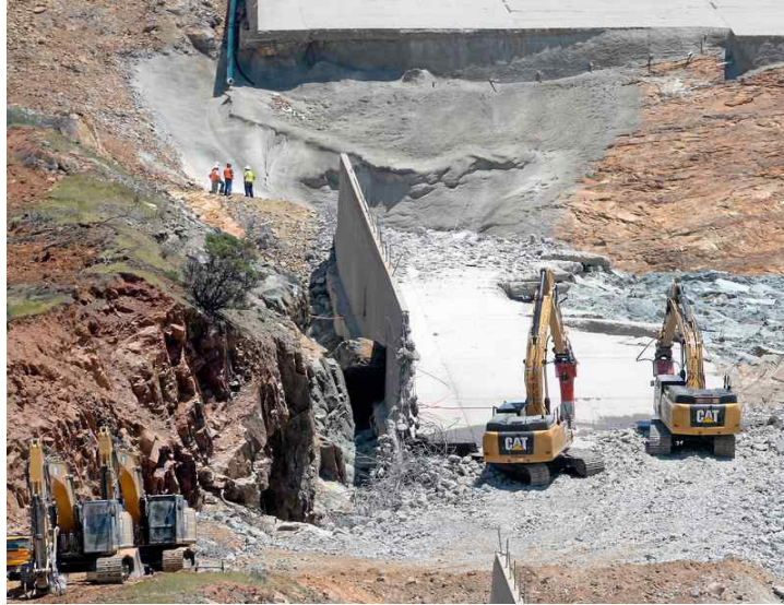
Heavy equipment works to break up remaining concrete on the lower part of the damaged main Oroville Dam spillway so a replacement can be constructed. (Bill Husa — Mercury-Register)
