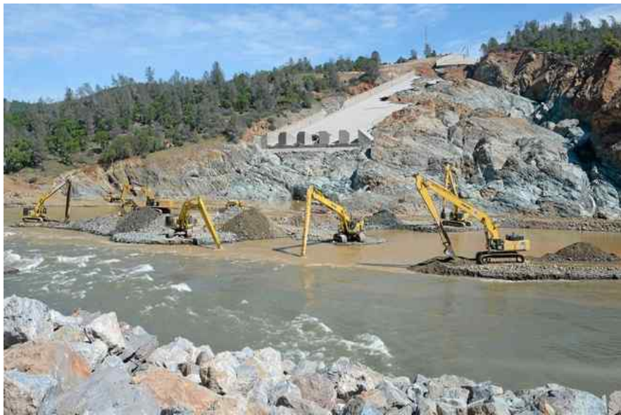
Excavators remove debris from the Diversion Pool below the main Oroville Dam spillway in this photo from March 29. Bill Husa — Mercury-Register
