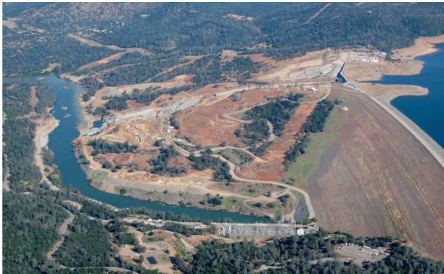
Oroville Dam and damaged spillways are seen Friday May 26, 2017
