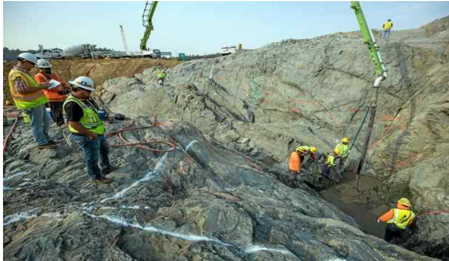
Concrete is pumped between rocks in the erosion area between the upper and lower chute at the Lake Oroville spillway on Monday. Ken James — DWR
