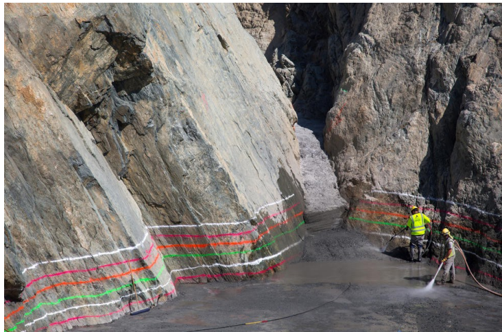
Loose material is washed from recently placed roller-compacted concrete (RCC) on the southeast side of the lower chute of the Lake Oroville flood control spillway. Photo taken July 24, 2017.
