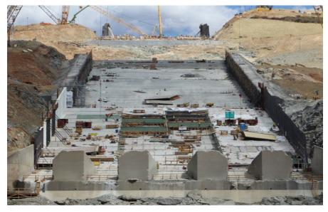
Crews set up concrete pours in a checkerboard pattern at Lake Oroville. Workers must wait four days for concrete to cure before pouring adjacent concrete. Millions of cubic feet of concrete will be poured before the project is completed.
