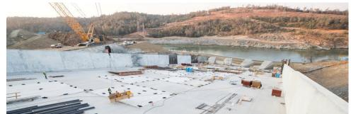
Crews continue placing rebar panels for the new sidewalls and structural concrete on the lower chute at the Lake Oroville flood control spillway in Butte County, California. Photo taken October 16, 2017. Ken James/ California Department of Water Resources
