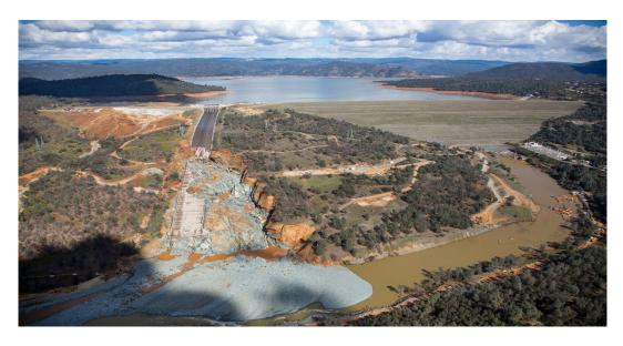
On 7 February this year, engineers spotted a hole in the concrete spillway of the tallest dam in the United States.
